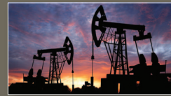
Oil & gas industry facilities.
